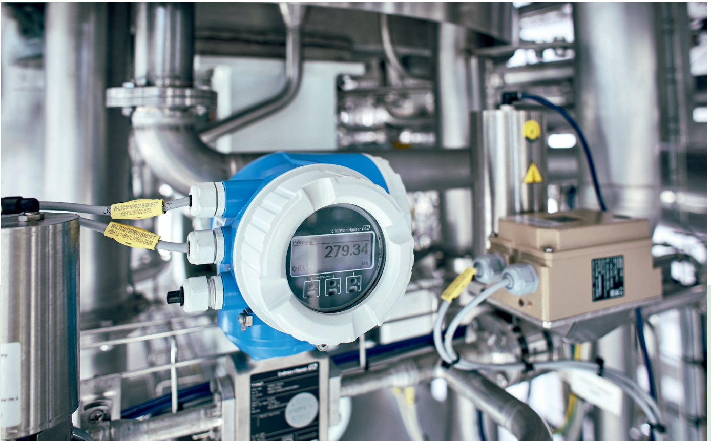
Smart sensors are the key to digitalization: The Proline 300/500 family of flowmeters features an integrated web server, WiFi and self-diagnostics systems.
